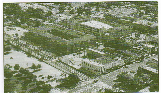
Downtown Plano light rail station
